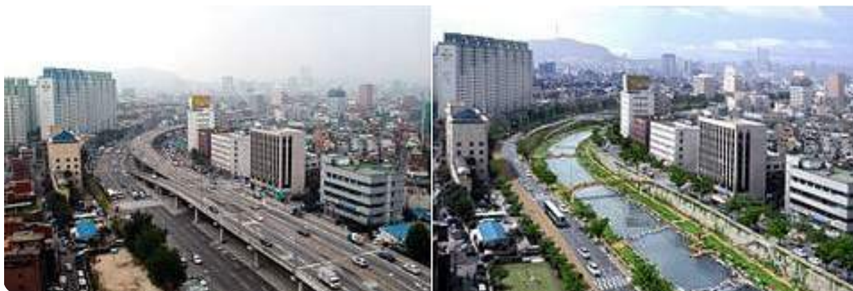
Transformation of the Cheonggyecheon River in Seoul, South Korea
